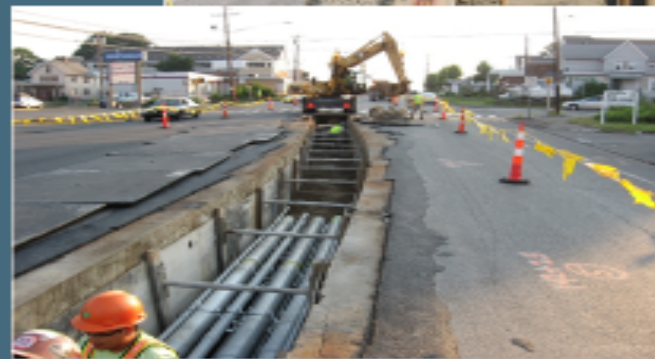
Northeast Utilities, Middletown – Norwalk 345 kV Transmission Project
