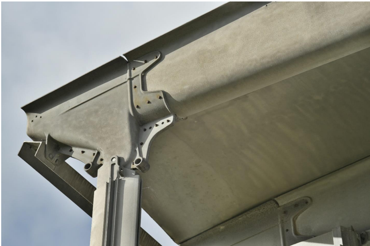
FIGURE 6: DETAIL OF CASTING FOR THE JOINT BETWEEN ROOF AND VERTICAL STRUCTURE FROM THE “PAVILION FOR THE CENTENNIAL OF ALUMINIUM” IN PARIS DESIGNED BY JEAN PROUVÉ
