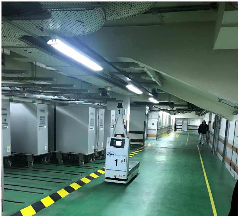
AUTOMATED DELIVERY OF PREPARED CONTAINER TO HOSPITAL SERVICES
