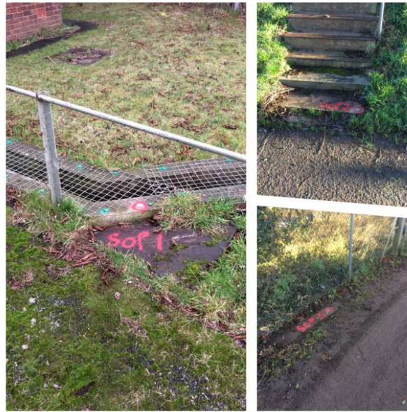
FIGURE 1: EXAMPLE OF SETOUT POINT (SOP) RECORDED BY A SURVEYOR
