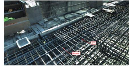
⑥ LEVEL 13 - Slab on Deck NTS
