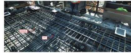
⑤ LEVEL 13 - Slab on Deck NTS
