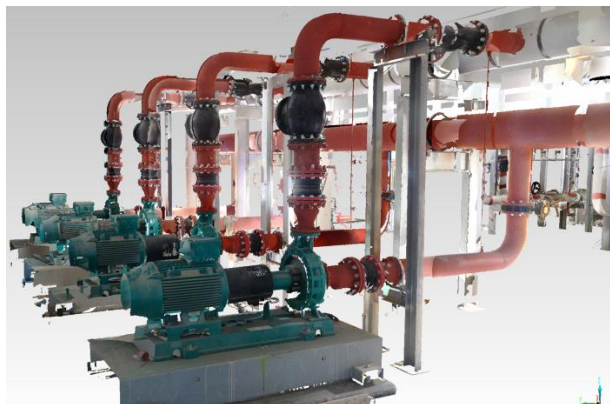
Pump Room Point Cloud Model
