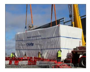
3D design and component standardisation were critical to the project's success. The modules were designed to be built in an off-site manufacturing facility. The off-site works included the fabrication of steel frame and fitting of the structural floor, installation of electrical equipment, such as UPSs, LV switchgear, battery racks, LV busbar installation to the perimeter of the modules, containment for LV submains, lighting, fire alarm and general services.
