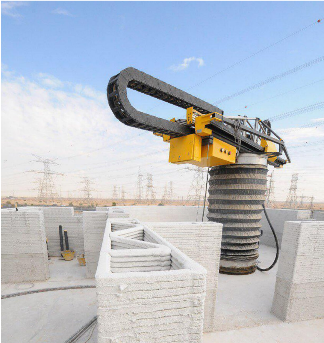
Apis Cor motion system for concrete extrusion https://www.apis-cor.com/
