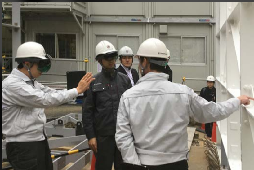
Checking the shape of the joint
