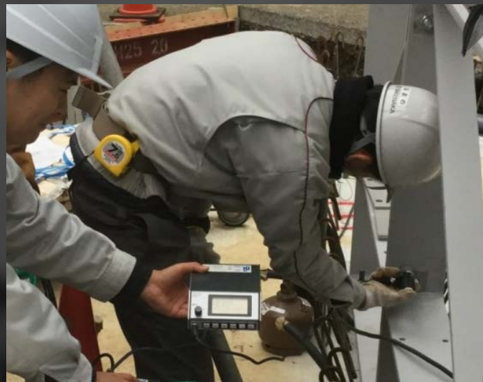
Checking steel material types
