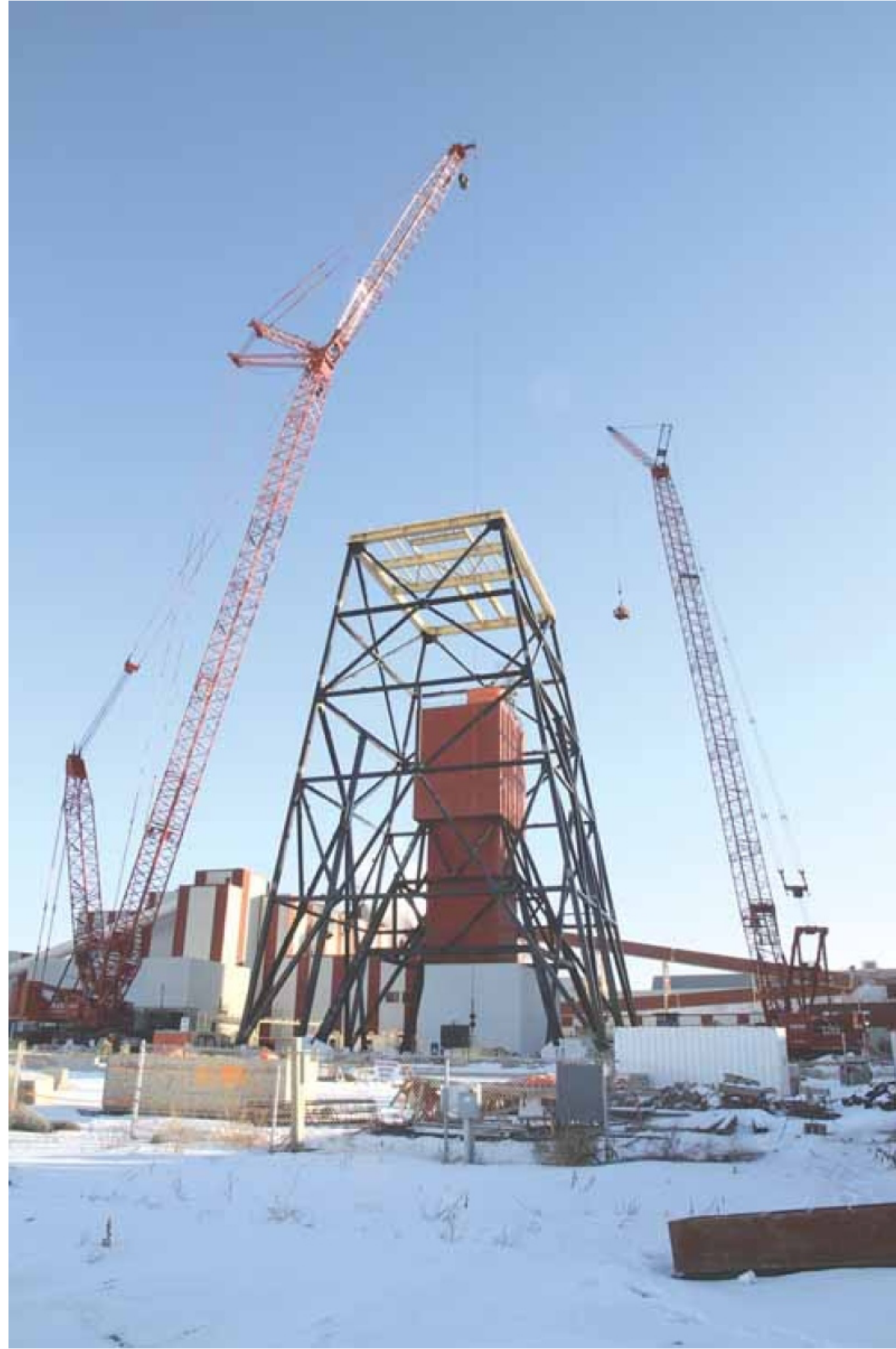
A new headframe for a second production shaft is built overtop of the current service shaft at the PotashCorp (Nutrien) Rocanville mine site- Retrieved from https://www.yorktonthisweek.com/news/local-news/potash-pink-gold-of-region-1.1516037
