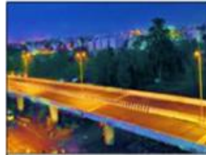
Heavy Civil Infra
