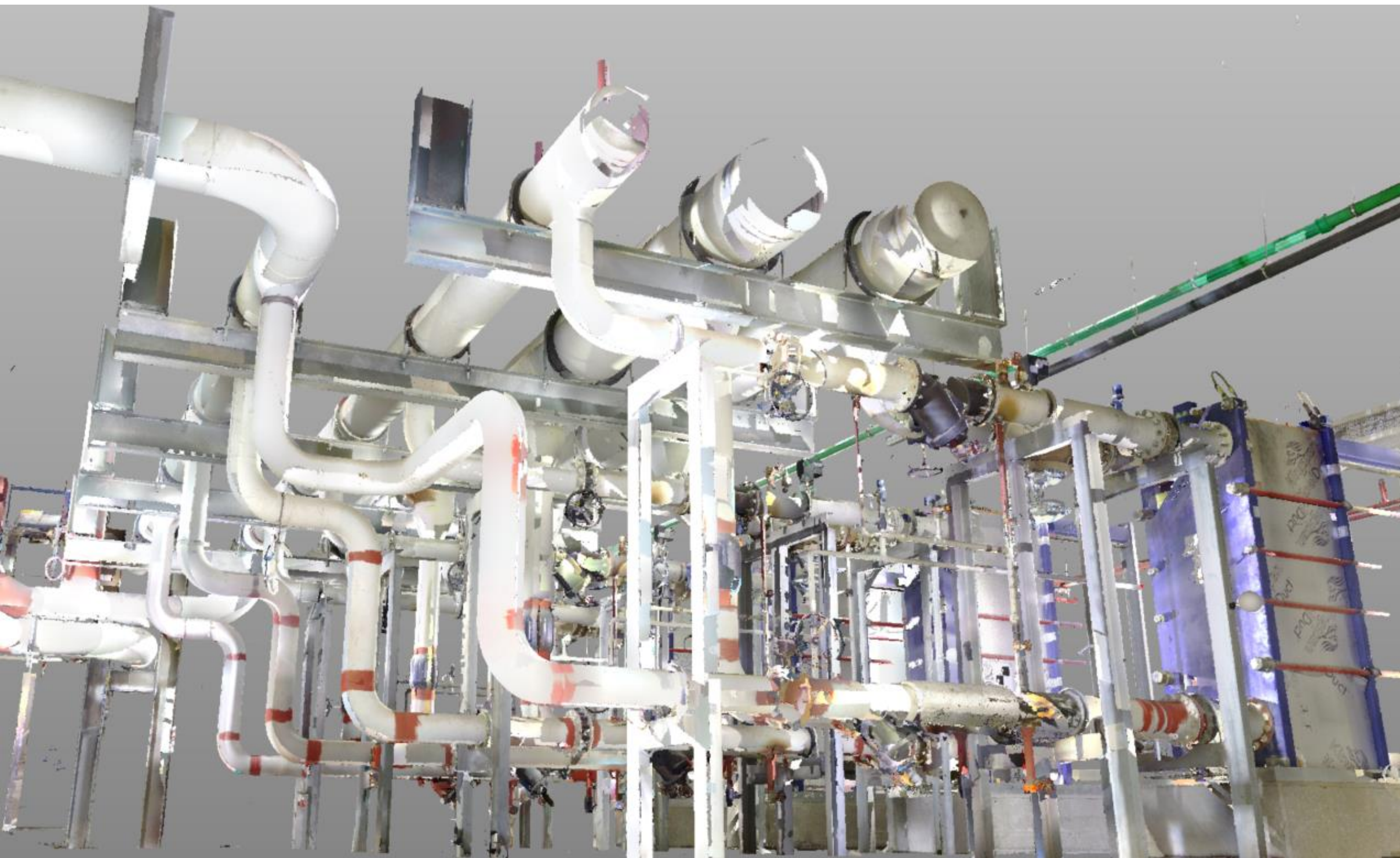
Chilled Water Pipes Point Cloud Model
