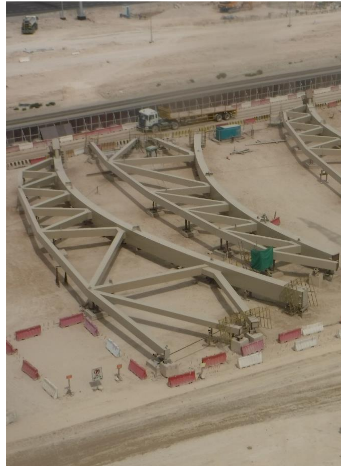
Steel Frame Assembly
