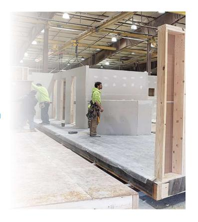
Increasingly manufacturing techniques are becoming commonplace within construction. Prefabrication and offsite manufacturing seeks to create construction components and assemblies in a controlled environment offsite before components transported to final destination for installation onsite. The aim is to reduce <u>material</u>, <u>overhead</u>, and <u>labour costs</u> relative to traditional construction techniques.
