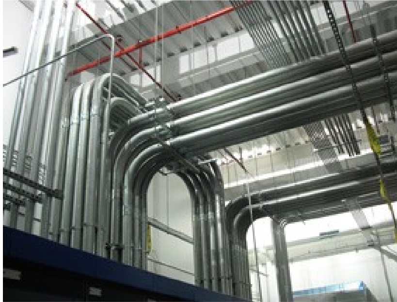
MULTI-TIERED TRAPEZE ASSEMBLY FOR CONDUIT
