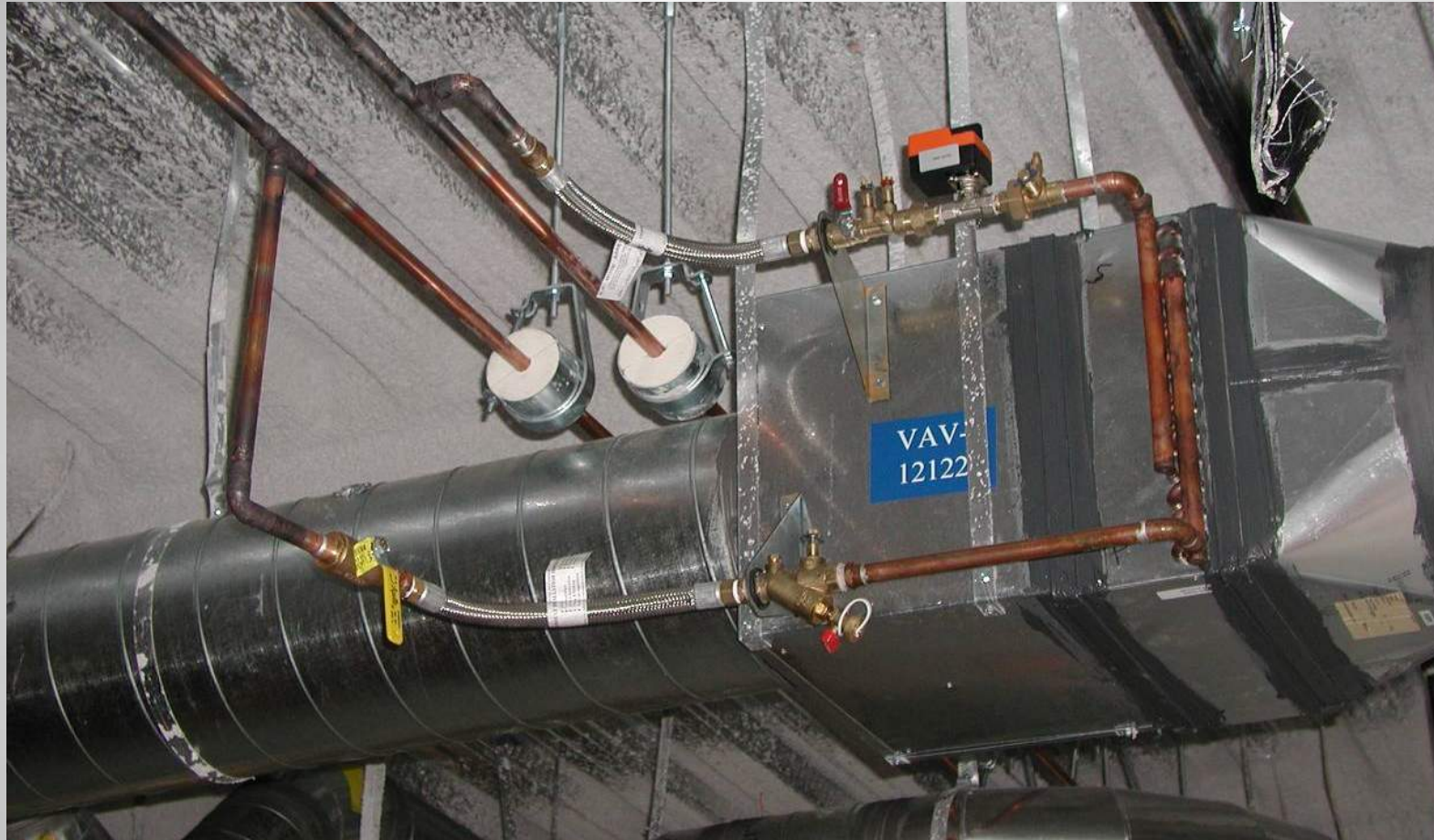
VAV assembly installed in field
