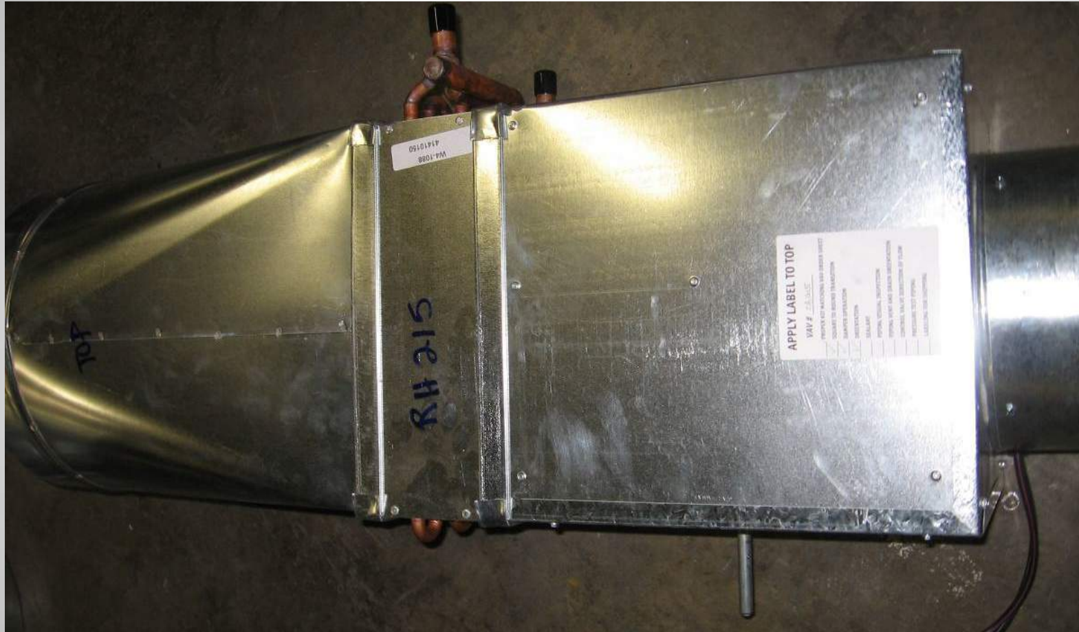
Attached assembled fitting to coil on VAV box.
