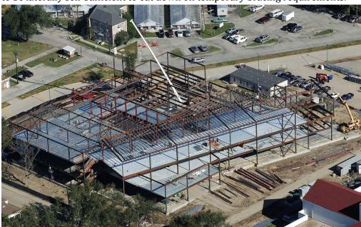
fabricator start early. Encourage the structural engineer to design phased portions to be laterally self-sufficient to cut down on temporary bracing requirements.
