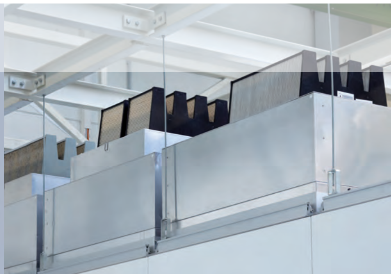
Filter Fan Units with AMC-filter (V-shape)
