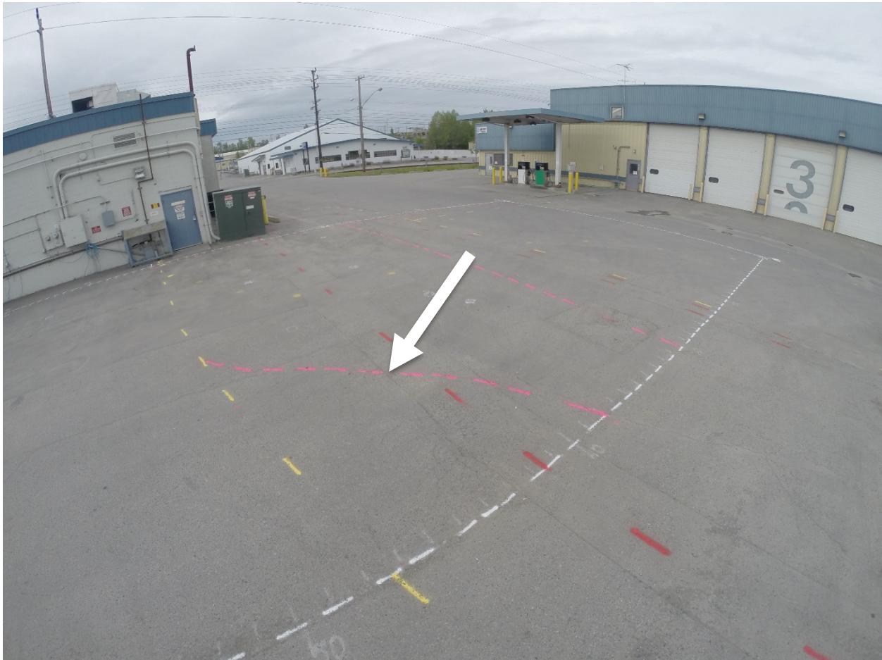
FIGURE 16. SOURCE AAML&P. GPR MARKS PAINTED ON A JOBSITE (PINK DENOTES UNKNOWN ANOMALY).
