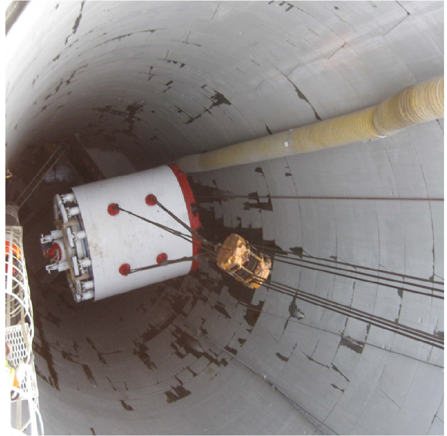
TBM being lowered in vertical access shaft
