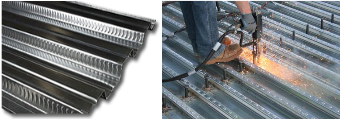
FIGURE 3: LEFT: COMPOSITE STEEL DECKING; RIGHT: WORKER WELDING STUDS THROUGH A COMPOSITE DECK.
