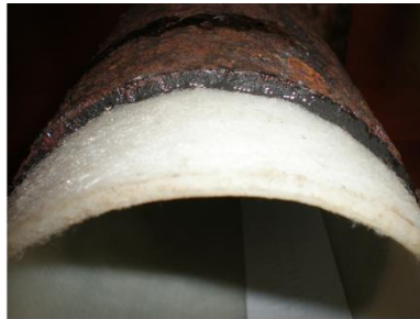
Cured-in-place pipe (CIPP) enables repair of deteriorating underground water/wastewater pipelines without expensive excavation. (Image: Craftsman Pipilining)
