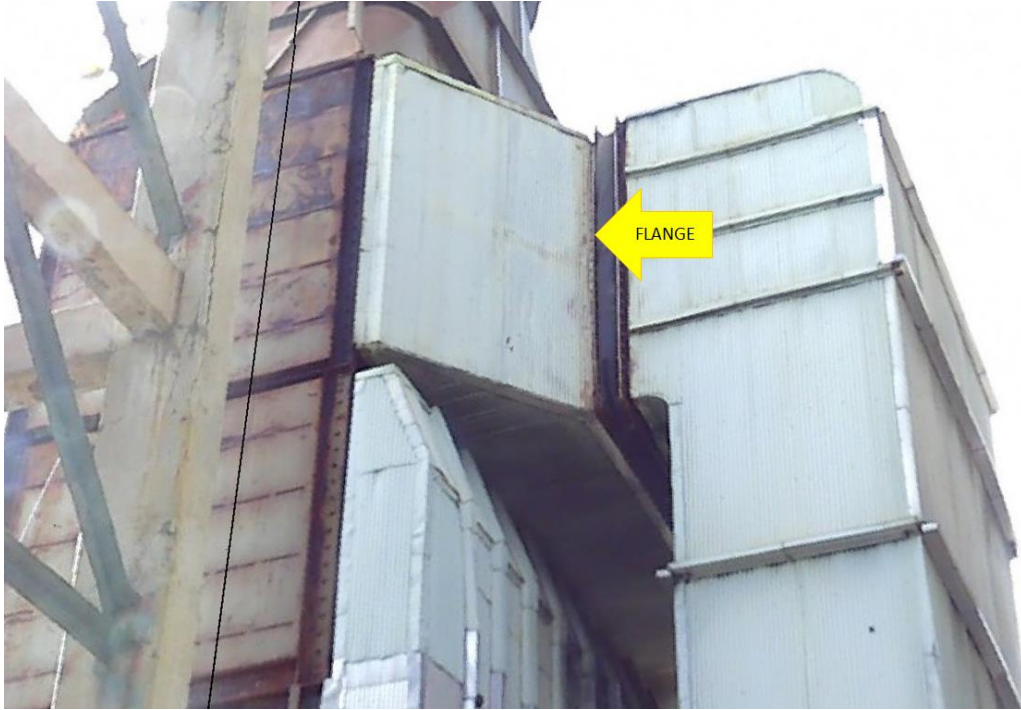
VIEW FROM THE SOUTH SIDE OF THE PREHEATER - LOOKING UP AT THE FLANGE CONNECTION AT THE HOT AIR OUTLET DUCT (PHOTO VIEW FROM LASER SCANNER)
