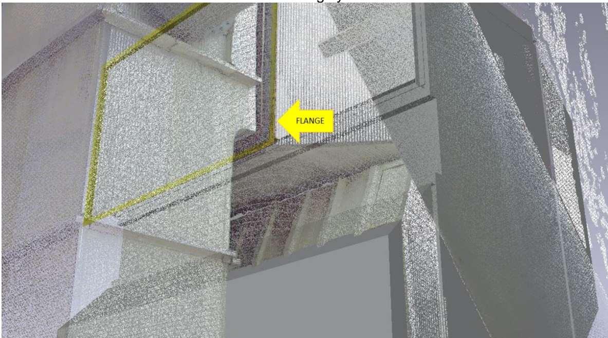
VIEW FROM THE NORTH WEST SIDE OF THE PREHEATER - LOOKING UP AT THE FLANGE CONNECTION AT THE HOT AIR OUTLET DUCT
