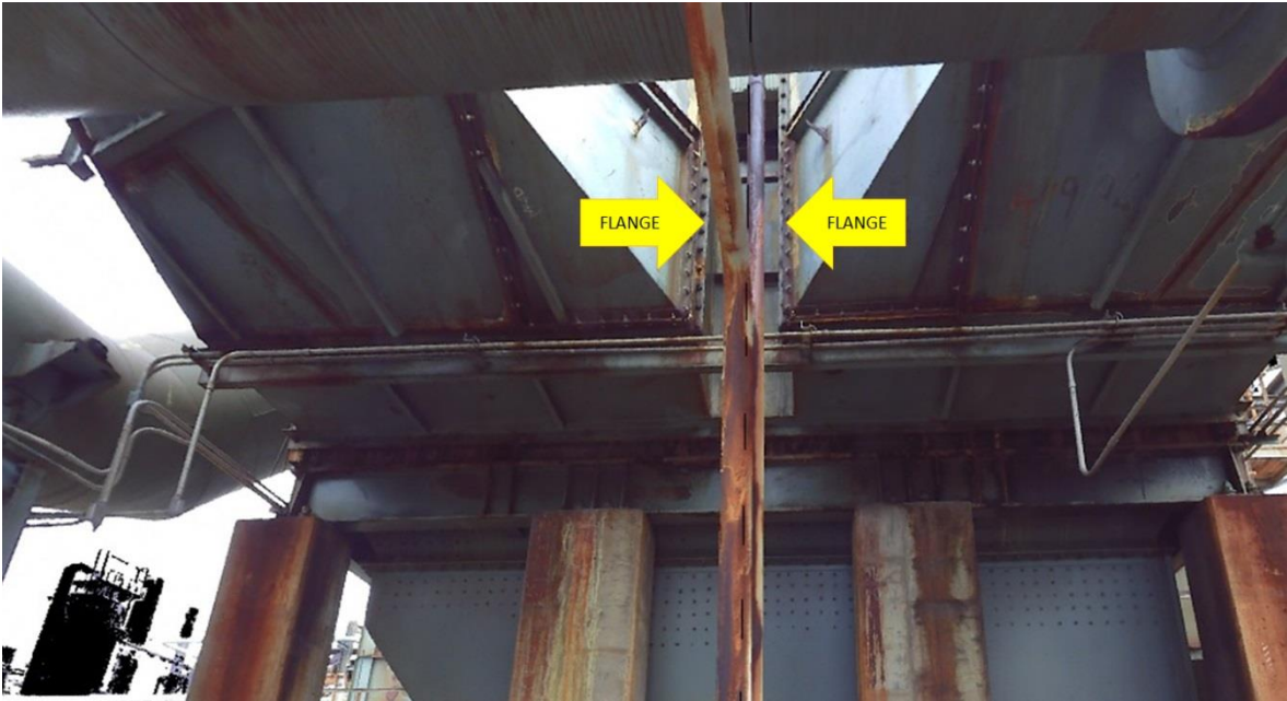
VIEW FROM THE WEST SIDE OF THE PREHEATER - LOOKING UP AT THE FLANGE CONNECTION AT THE COLD AIR INLET DUCT (PHOTO VIEW FROM LASER SCANNER)
