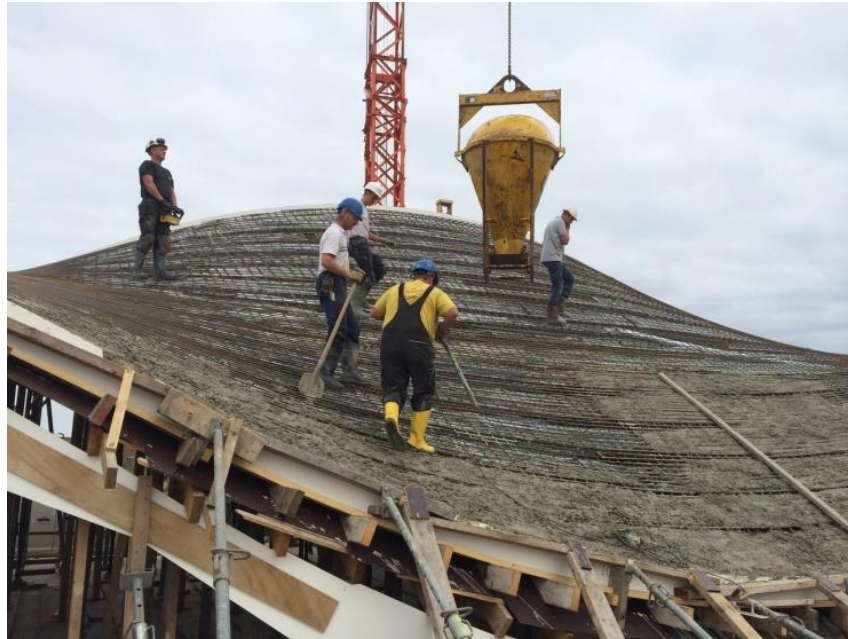
POURING THE CONCRETE ON THE COUCH. APPLYING A SIMPLE GRID OF REINFORCEMENT ON A COMPLEX SHAPE DOES NOT INCREASE COMPLEXITY OF CONSTRUCTION.
