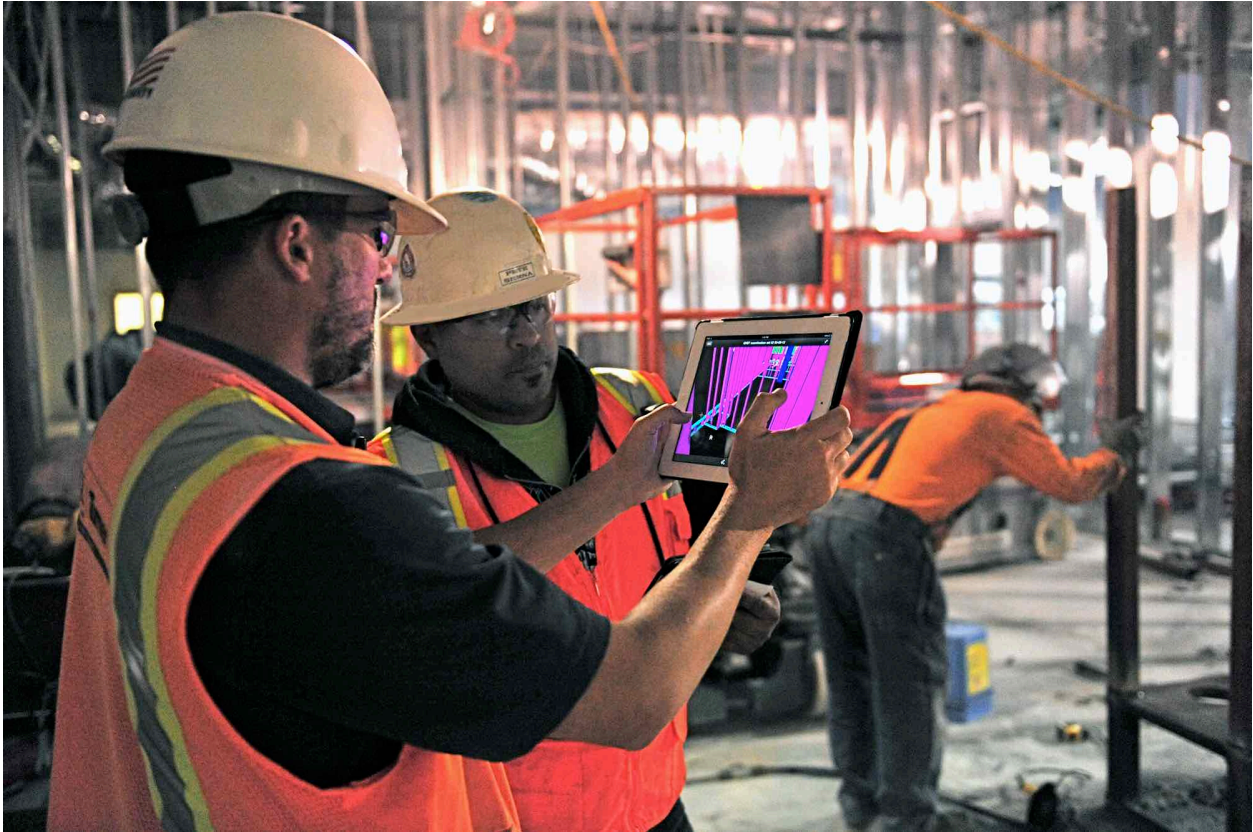
FIGURE 24. FIELD FOREMAN LOOKING AT BIM FOR FRAMING AND IN-WALL UTILITIES DETAILS. LICENSED BY THE REGENTS OF THE UNIVERSITY OF CALIFORNIA ON BEHALF OF ITS UCSF MEDICAL CENTER; COURTESY OF DPR CONSTRUCTION; COURTESY OF MIRROR MIRROR DIGITAL MEDIA, INC.
