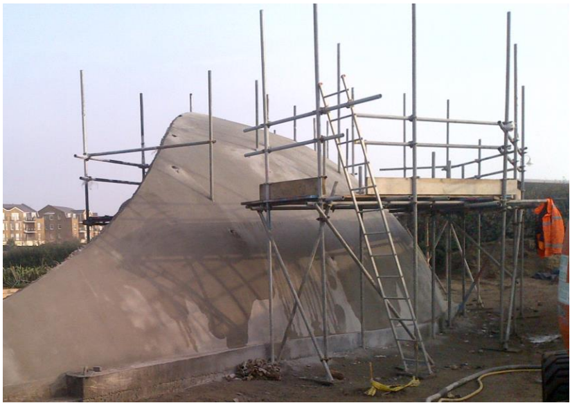
Image of the temporary steel poles penetrating the concrete form.
