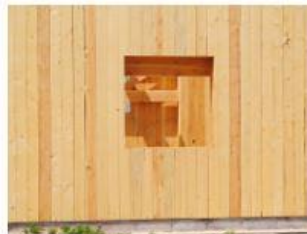
Interlocking CLT from beetle kill pine
