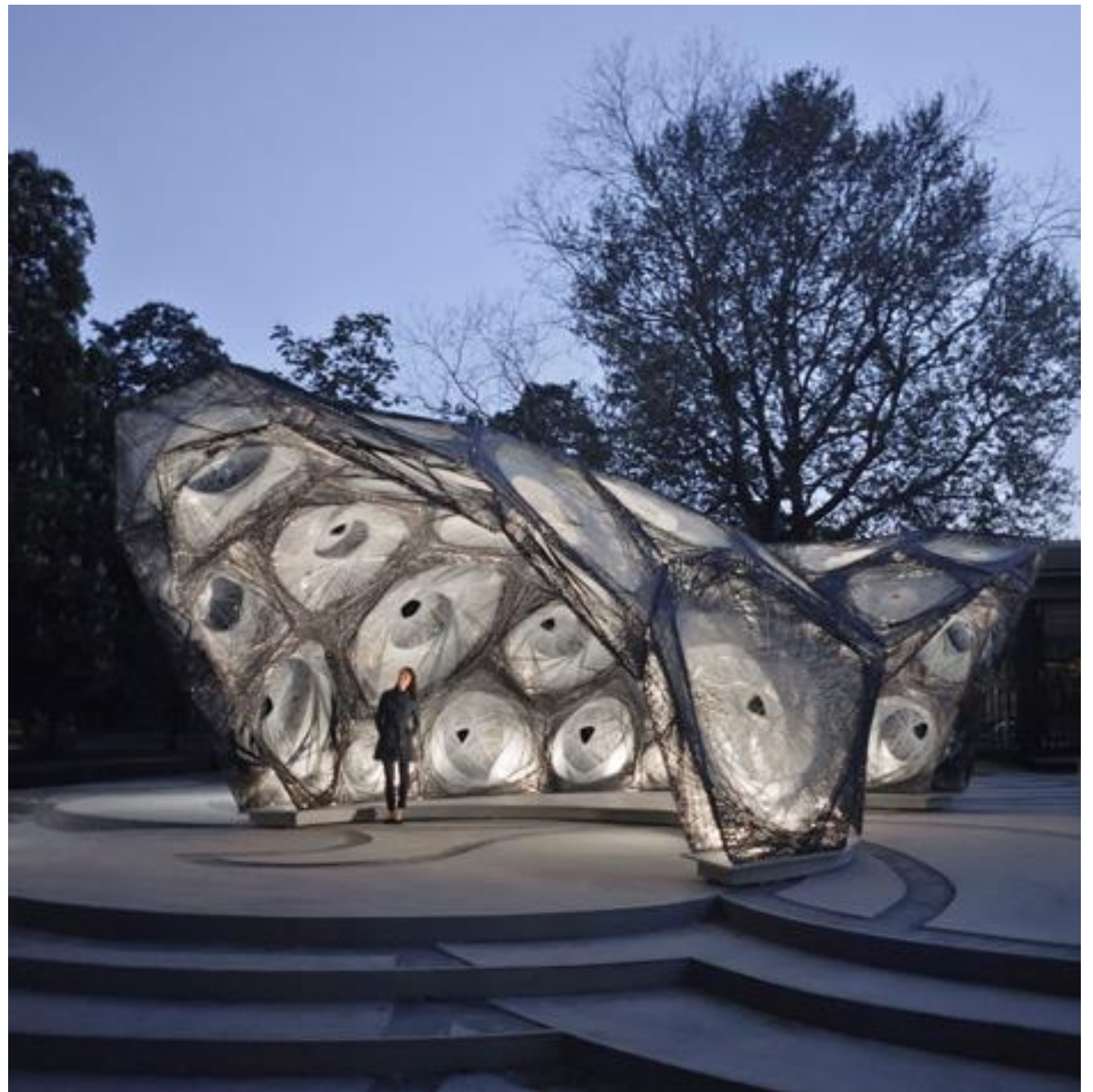
Stuttgart University Pavilion made from carbon fiber by robots
