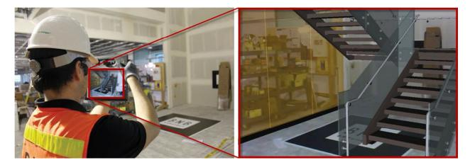
Additional uses are projected to incorporate systems like Google Glass to overlay data (model and text) for visualization at any phase of design or construction. Imagine the plumbing assembly placed virtually in a building showing the plumber not only where the piping is to be routed, but the specifications, and any other pertinent information.
