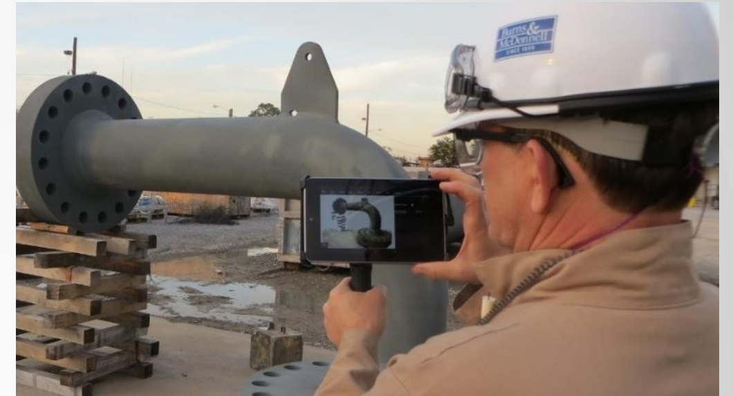
Spool verification with the DPI-7 at an oil refinery in New Orleans
